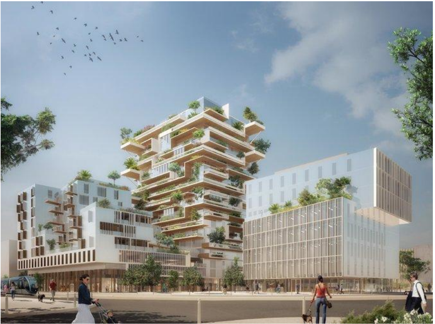
The Hypérion, a project commissioned in Bordeaux, France. Credit Jean-Paul Viguier et Associés
